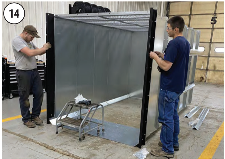
Bolt the tailgate support channels to the side panels & floor plate with (11) 5/16"-18 x 1" flange screws & 5/16"-18 locknuts each.
