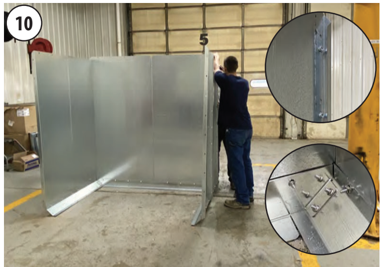
10 Stand up the front panel assembly and bolt one side panel assembly to each end with (11) 5/16"-18 x 1" flange screws & 5/16"-18 locknuts.
