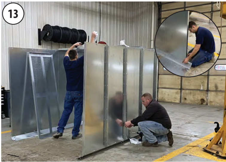
Repeat steps 6 - 12 for the remaining side & top panels. Note: The last side panels will bolt to the floor plate instead of a floor channel.
